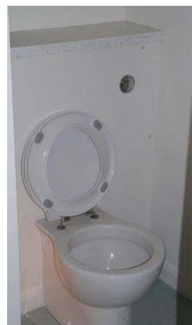
Smaller toilet uses less water; has dual action flush; note recycled plastic worksurface material (old mobile phones!)
